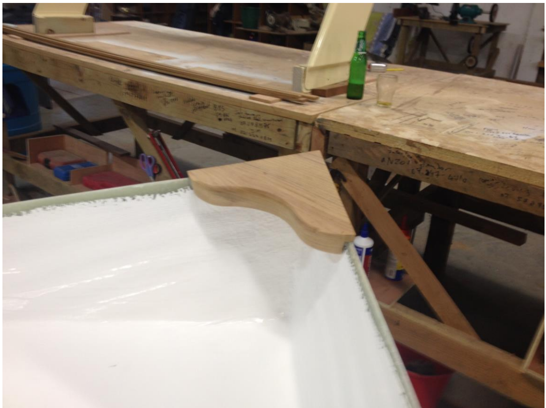
Installation of the teak woodwork begins.
